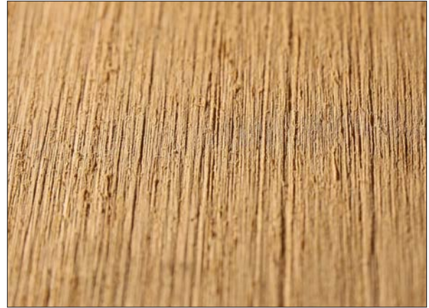
This is a close-up image of a floor that has been 1st cut with 40 grit.
