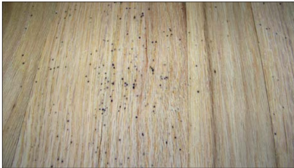
Do not sharpen scrapers on raw wood when using waterborne finishes. The filings may cause rust spots or black spots in the finish.
